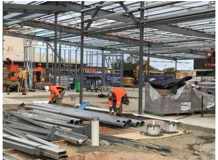
Above: Construction of the non clinical services building and associated works is on-track with internal and external steel wall framing underway as well as the installation of building services including electrical, water, fire and air-conditioning.
