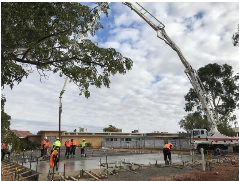
Pictured (above): The concrete slab of the temporary Paediatric Unit was poured in late April (right) installation of new stormwater and sewer services along Warrambool St is nearing completion.
