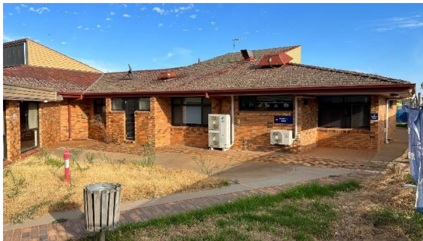
Figure 4: Building 24 Children's Ward
