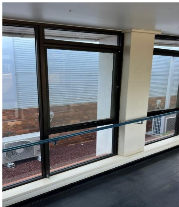
Figure 2: Building 23 Connection Walkway
