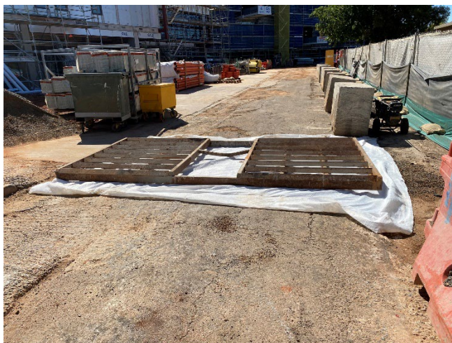
Construction site access with geotextile under rumble grid. Sediment fencing along the southern boundary fence. Sand bags visible to keep the sediment fencing in contact with the ground.
