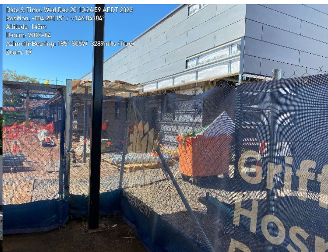
Orange waste skip bin and sediment fencing along the perimeter fence along the north-western boundary.
