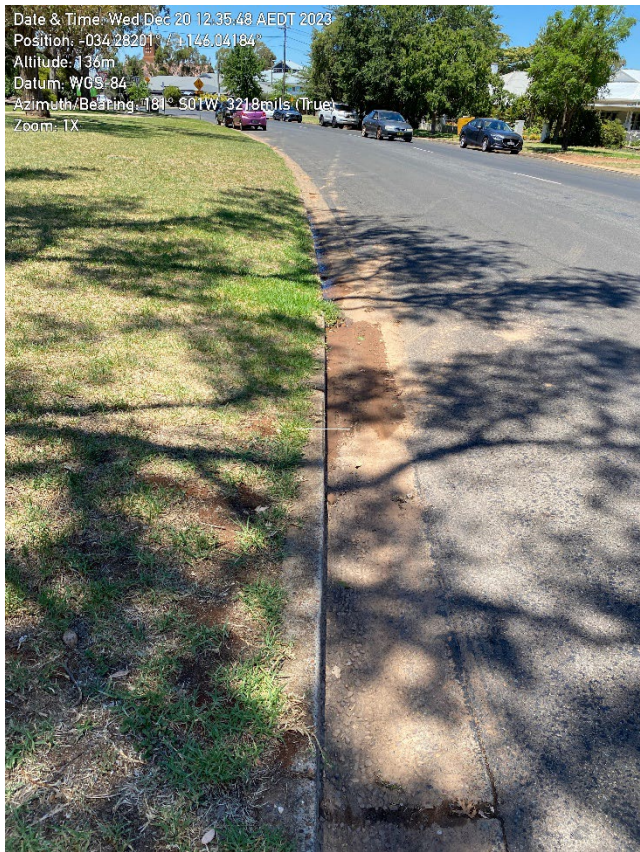
Sedimentation in gutter of Animoo Avenue, down-gradient from the site access.
