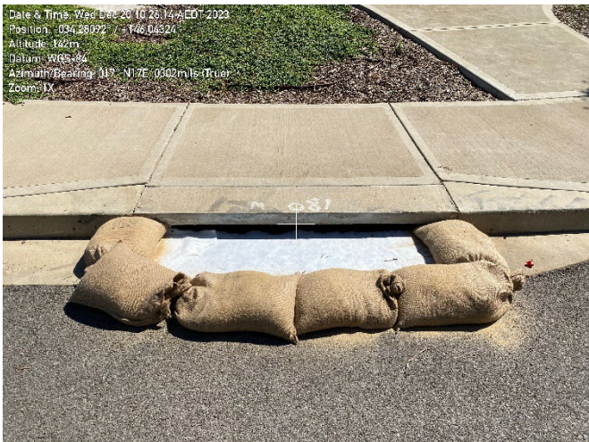
Drain protection with clean geofabric and sand bags.
