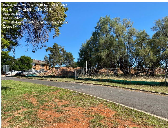
Sediment fencing around the contractor parking area and spoil storage area.
