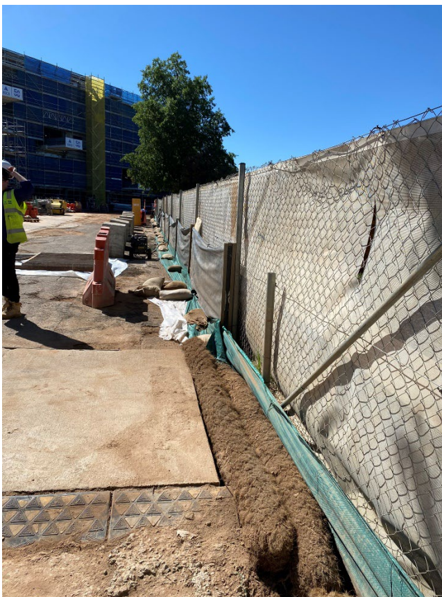
Maintained sediment fence and coir logs at site access, adjacent to southern boundary.
