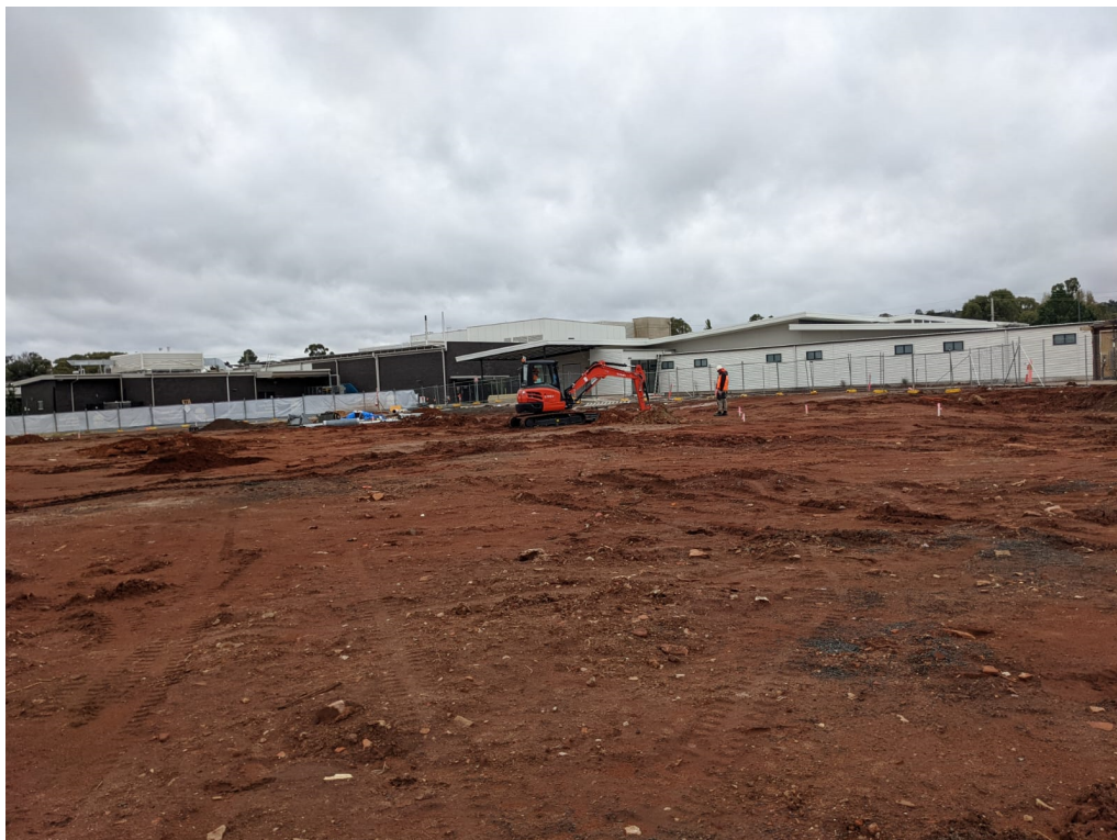
Photograph 4: View of general site conditions, looking north west.
